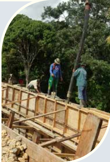
PDRC Workers involved in the construction of Retaining Wall at Assiah Trace
