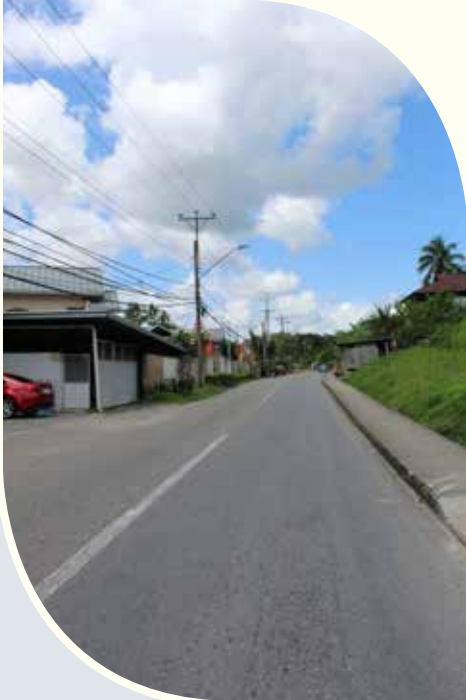
Resurfaced New Colonial Road from Barrackpore to Borde Narve
